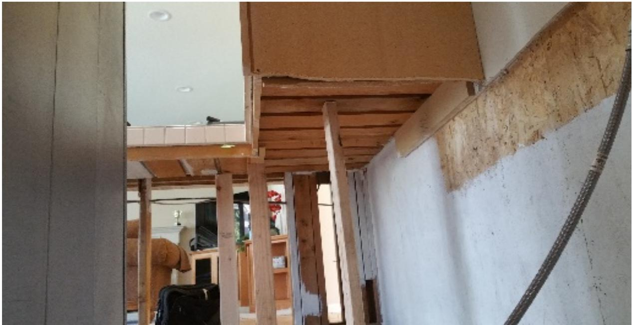
Example of removed kitchen cabinets where the countertop is salvageable. Lower “new” cabinet boxes and “original face frame and cabinet doors” must match the 30-year old cabinets.
